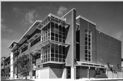
The Langston-Brown School and Community Center uses extensive interior daylighting with sunshades to control heating from the hot summer sun. Two large cisterns capture rainwater from the roof, which can be used for irrigation around the building. During construction, over 80% of construction debris was recycled.
