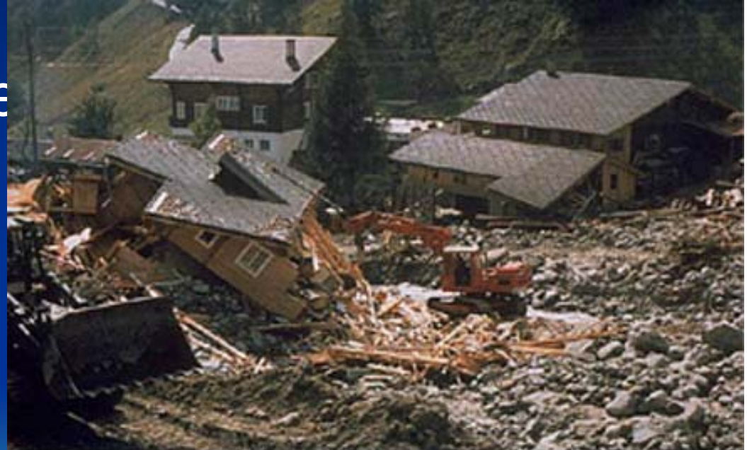
Houses undermined by melting Permafrost
